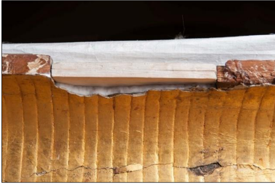
Figure (10) temporary consolidation of a large void with balsam wood
