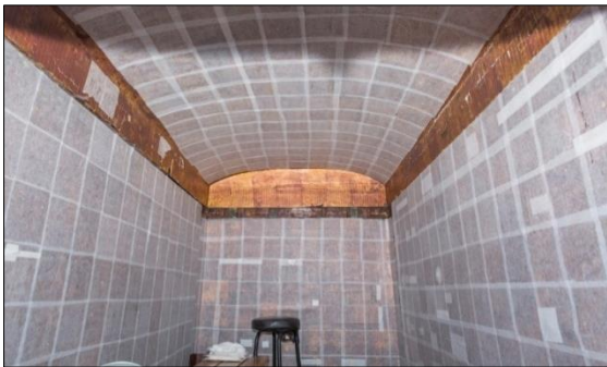
Figure (11) facing performed on the interior of the shrine using 9g. tissue paper and 1% Klucel G. w/v in ethyl alcohol
